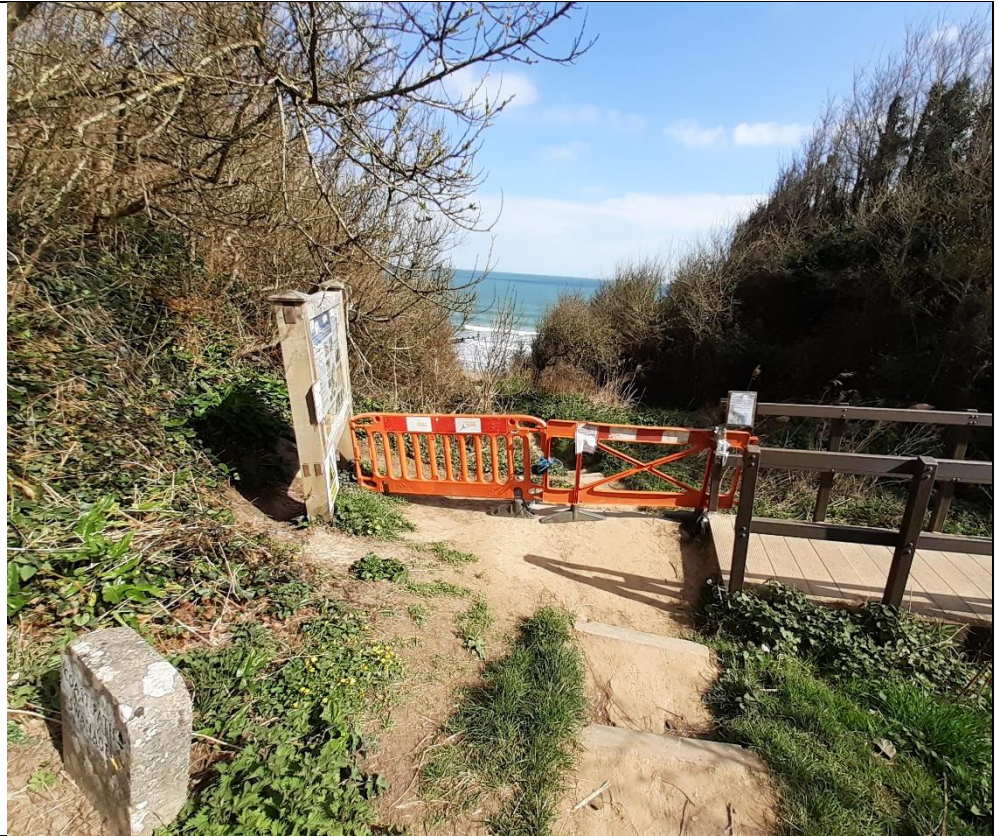
Site of work – between barrier and sea
