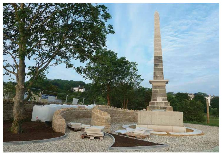
The reconstruction of the original Prince Albert Memorial is now reaching its finale with only the finishing touches - the stone facing of the plinth, the railings with corner supports, paving and surfacing of the paths, benches and planting - needing to be completed.
