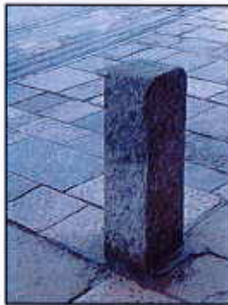
Image 12: Stone bollard on The Square with no tonal contrast with surround
