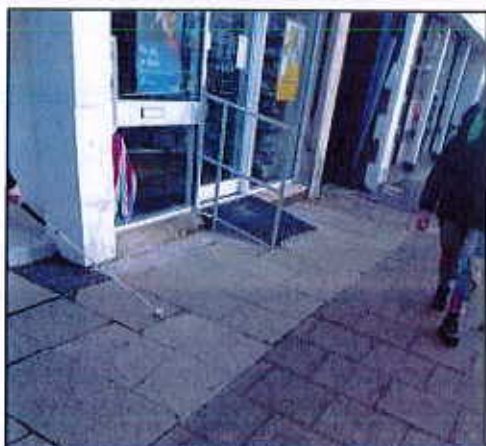
Image 9: Shop entrance with ramp for low riser
