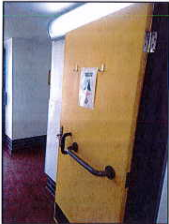
Image 19: Door to accessible toilet with high hooks meaning you have to stand to be able to hang any clothing or items
