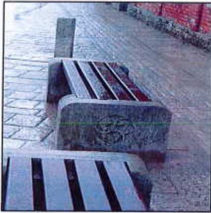
Image 14: Low level seating with low contrast to the surroundings and no arms rests
